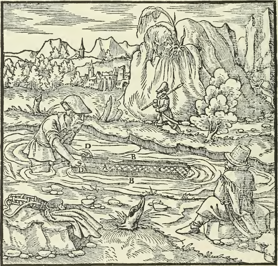
A—PLANK. B—SIDE-BOARDS. C—IRON WIRE. D—HANDLES.
